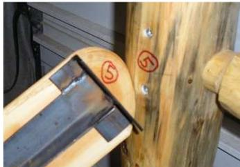
5. Bolt the side rails into their respective places, halfway only, do not tighten yet. Once all the bolts are started half way, go ahead and tighten them SNUG, do NOT overtighten.
